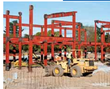
Student Services Center construction
