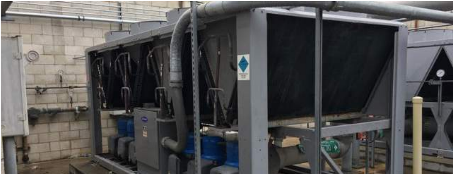
Replacement of the chiller units at LVC
