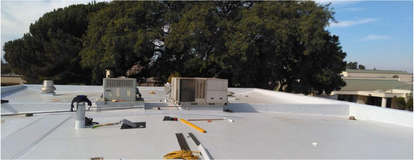
Building H Roof Replacement
