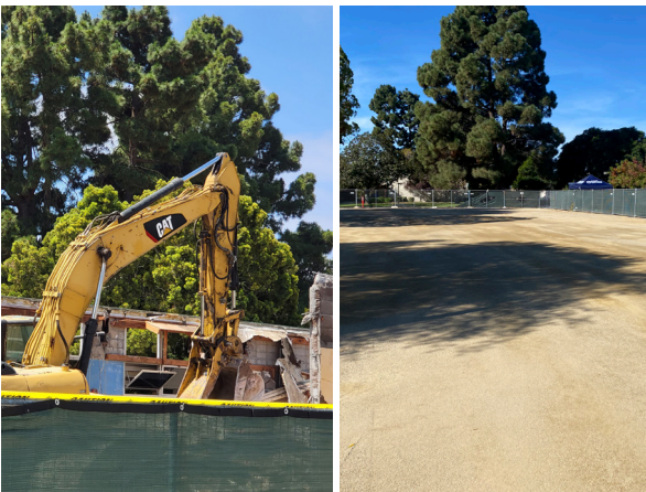
Buildings E & F during and after demolition.
