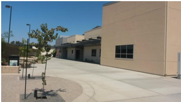
Building O-100 from Courtyard
