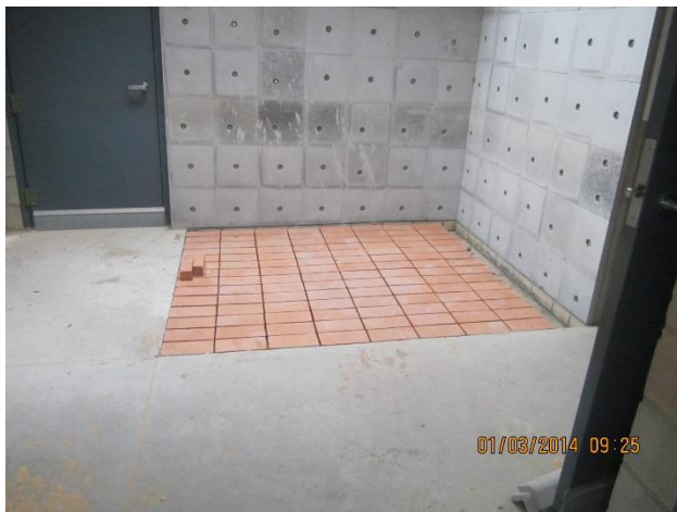
Fire Brick at the Burn Bldg.
