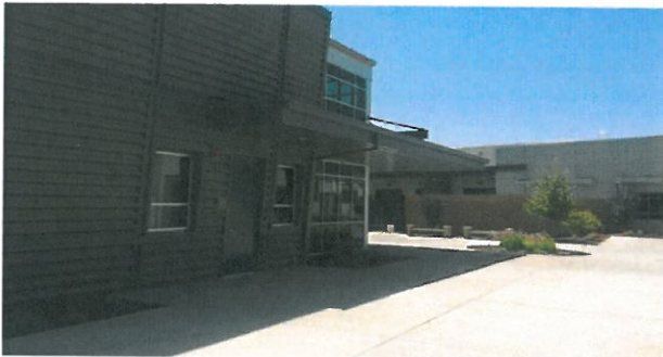
Building O-100 at Entry
