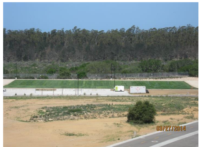
Sod at Running Track
