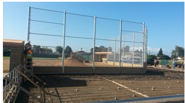
Softball Field Progress
