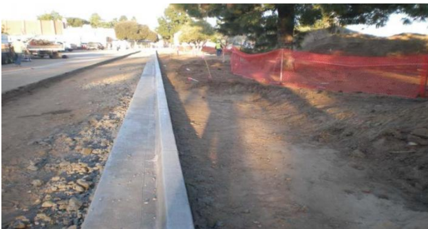
Curb and gutter installation at south side of greenbelt area
