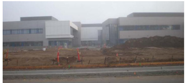
Preparation for concrete sidewalks at greenbelt area.
