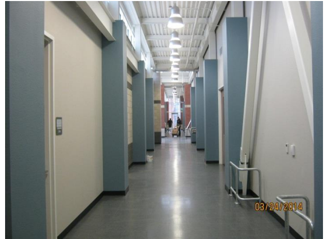
Admin. Bldg. – VCT flooring
