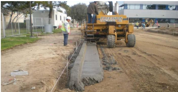
Curb and gutter construction along west side of greenbelt area
