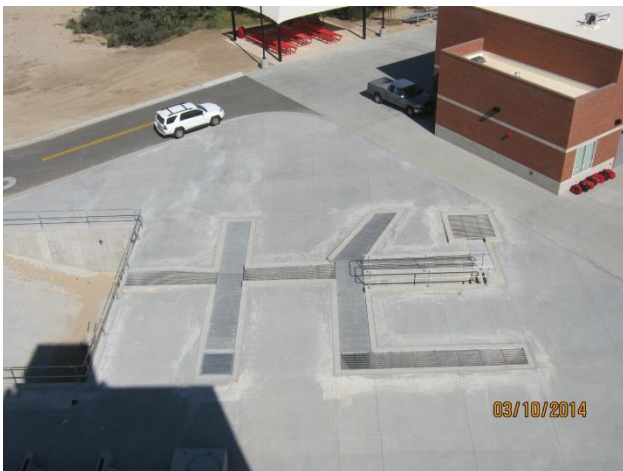
Trench Rescue/ Confined Space with safety rails
