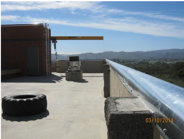
Fire Tower – Jib crane and parapet cap
