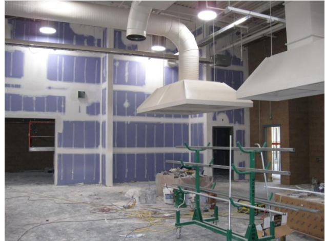
Drywall installation at Building 0-200 Welding Lab
