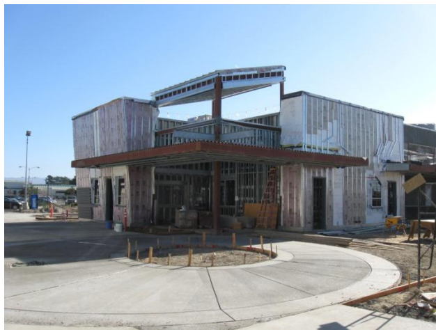
Northwest corner of Building O-100
