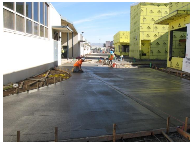
Flatwork installation between Buildings O & O-200
