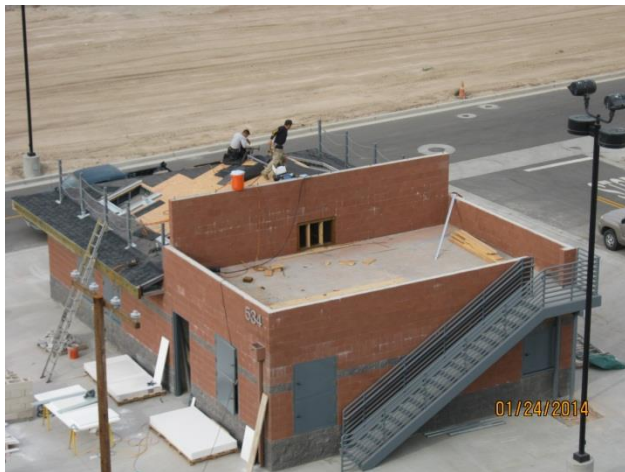
Class A Burn Bldg. – Comp shingle roof installation
