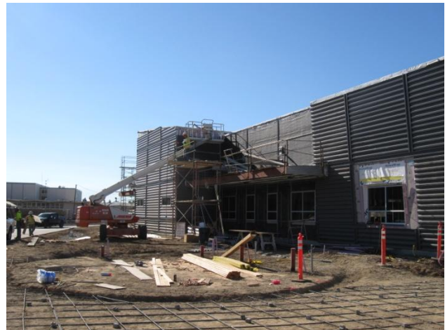
Metal siding installation at Building 0-100
