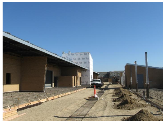
Rebar & formwork at Industrial Tech Yard
