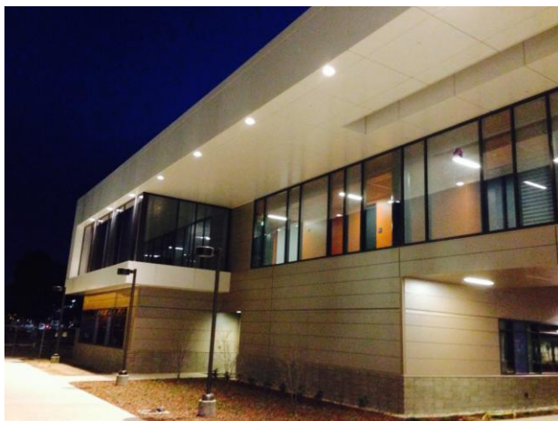
Building A2 and related exterior lighting
