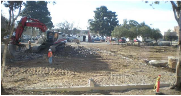
Cleared site of former building A
