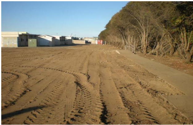
Cleared site of former buildings T, U, V and X
