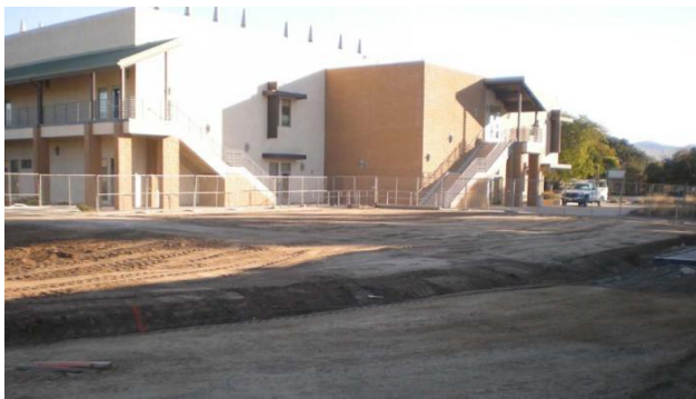
Cleared site of former building N2
