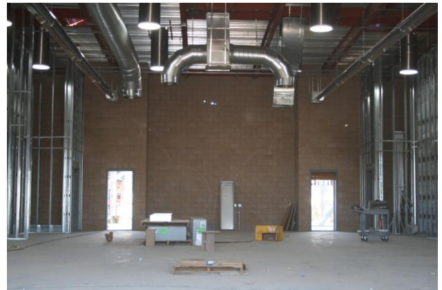
Metal Framing & Mechanical Installations @ Welding Lab (O-200)
