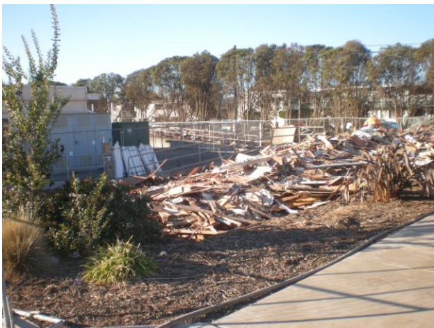
Building Demolition in progress.
