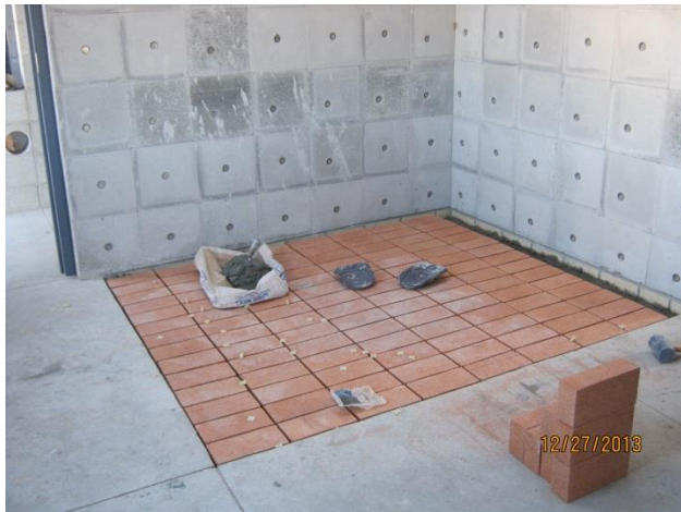
Class A Burn Bldg. – fire brick installation
