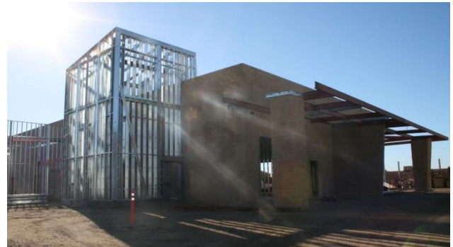
Metal Framing @ South College Drive Entrance (O-200)
