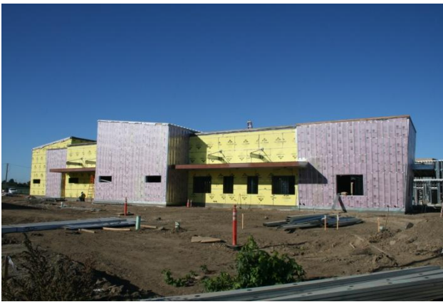
Industrial Technology Building (O-100)
