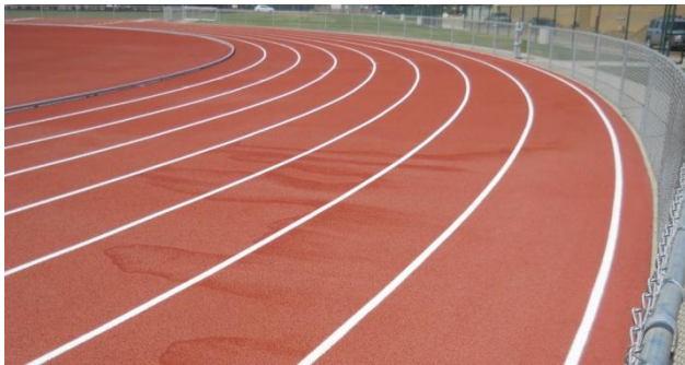
View of Track Looking North – Track Curbing & Striping
