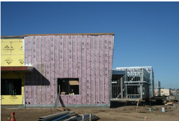
Admin. Building O-100 (O-200 Classrooms in Background)
