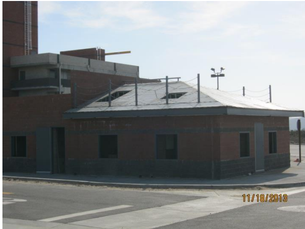
Class A Burn Bldg. – Metal decking
