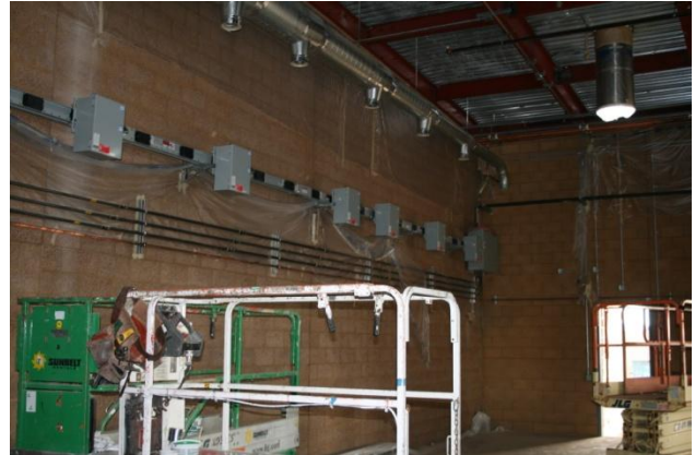
M-E-P Rough-In at Building 0-200 Welding Lab 3
