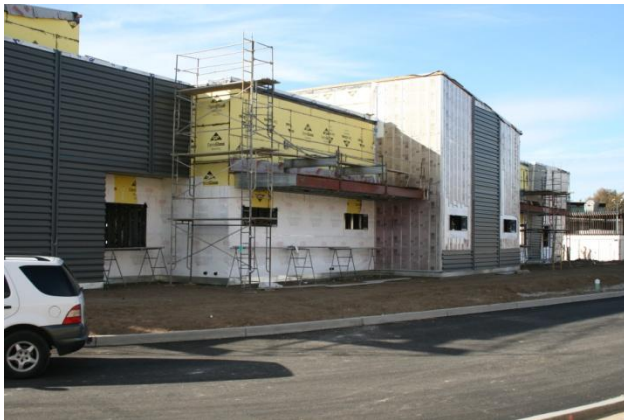
Moisture-Resistive Barrier Installation at Building O-100
