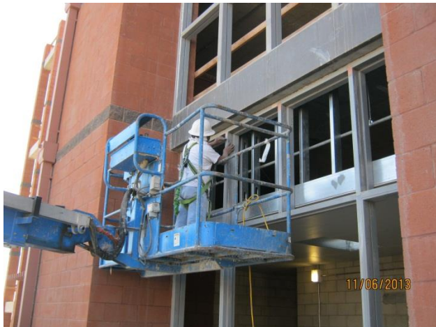
Fire Tower – Hollow metal frame painting
