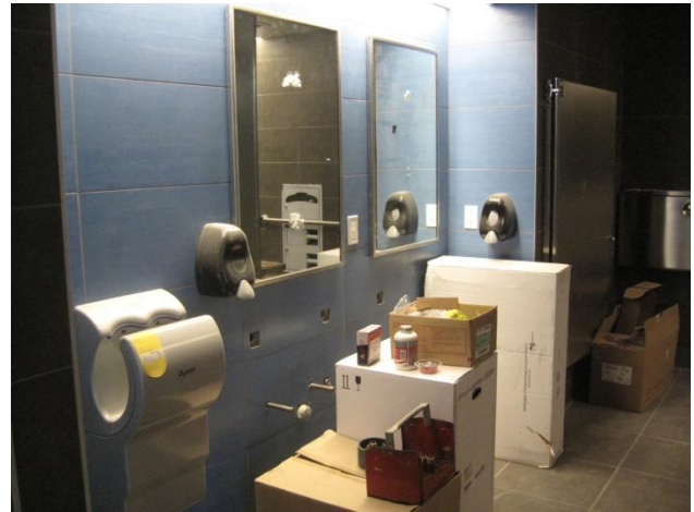
Building B Restroom tile and mirror installation
