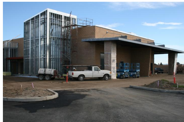
West end of Building O-200 - Enology Lab
