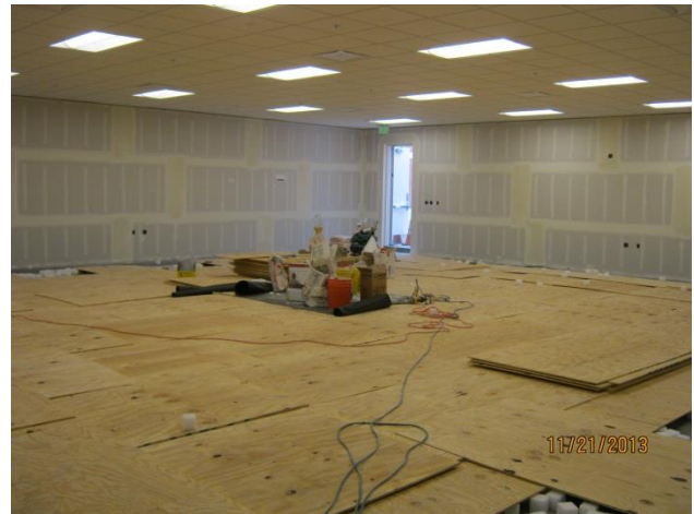
Admin. Bldg. – Tatami mat installation
