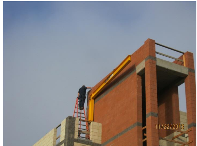
Fire Tower – Jib crane installation
