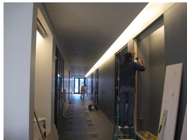
Tile at and touch-up paint at Building B corridor
