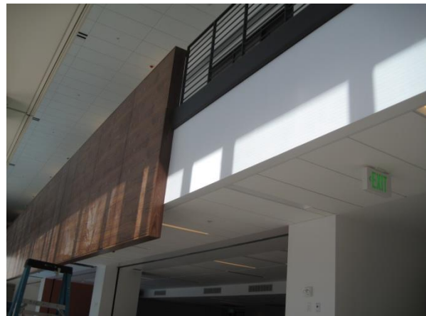
Completed wood panel installation
