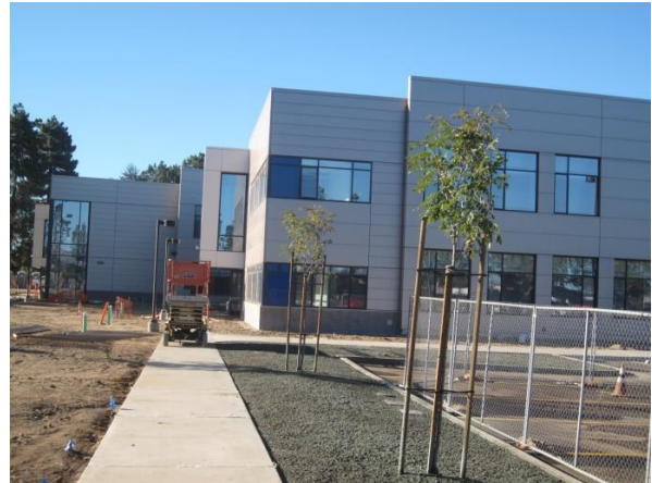
North Parking Lot hydroseed and tree installation
