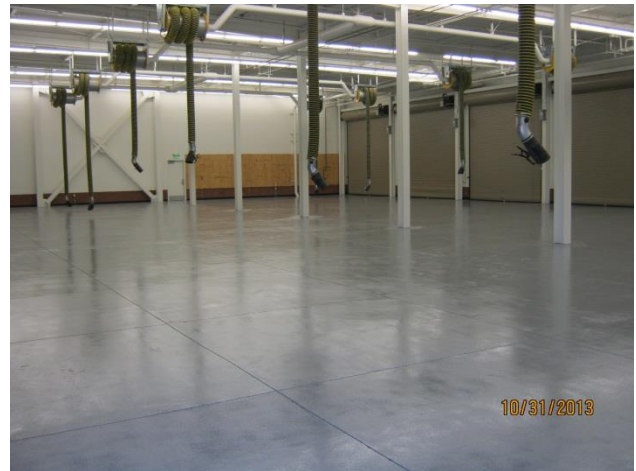
Vehicle Storage. Bldg. – Concrete Epoxy Placement
