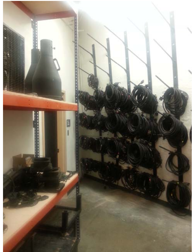
New Storage at Lighting Shop
