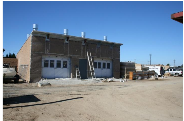
Preparing Paint Booth Enclosure Building for Exterior Paint
