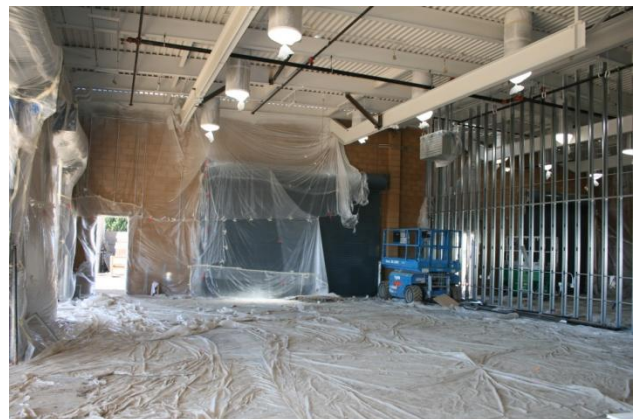
Auto Body Lab Interior Painting @ Underside of Metal Roof Deck
