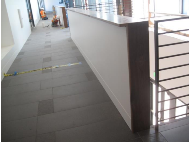
Interior tile at second floor.
