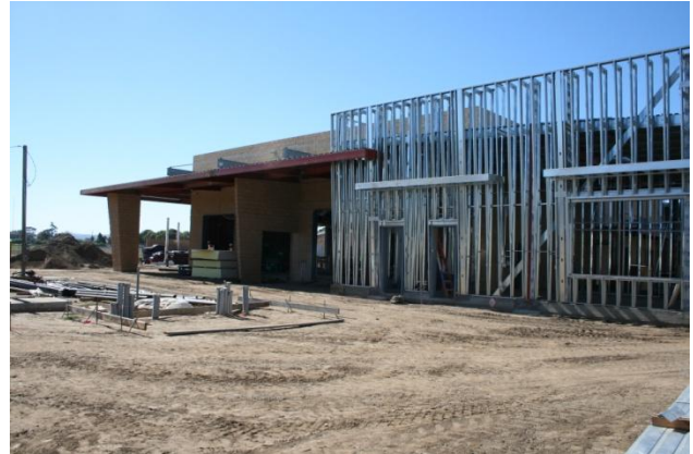
Industrial Tech Lab Building (O-200)
