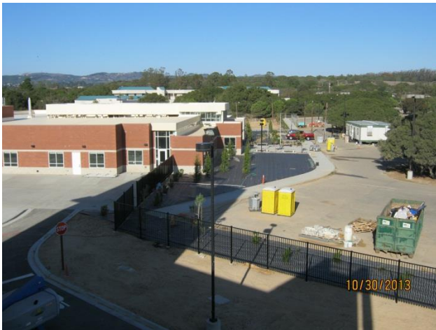
Administration Bldg. – Main entryway
