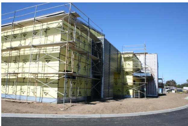
Scaffolding for Lath & Plaster Installation at O-100
