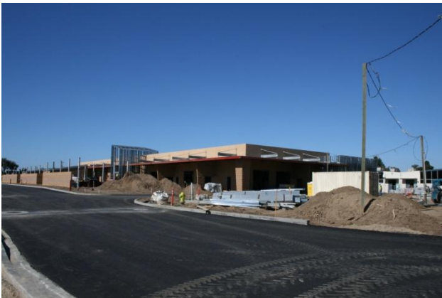
Industrial Tech Lab Building (O-200)
