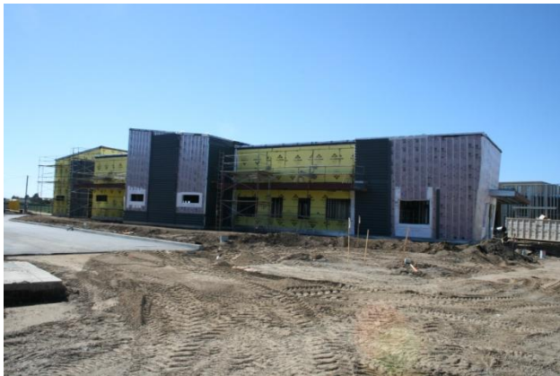
Industrial Technology Building (O-100)
