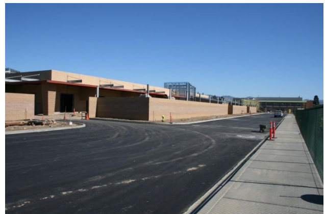
Loop Road Paving
