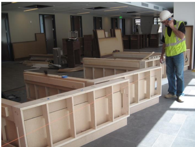
Service counter installation at Financial Aid.
