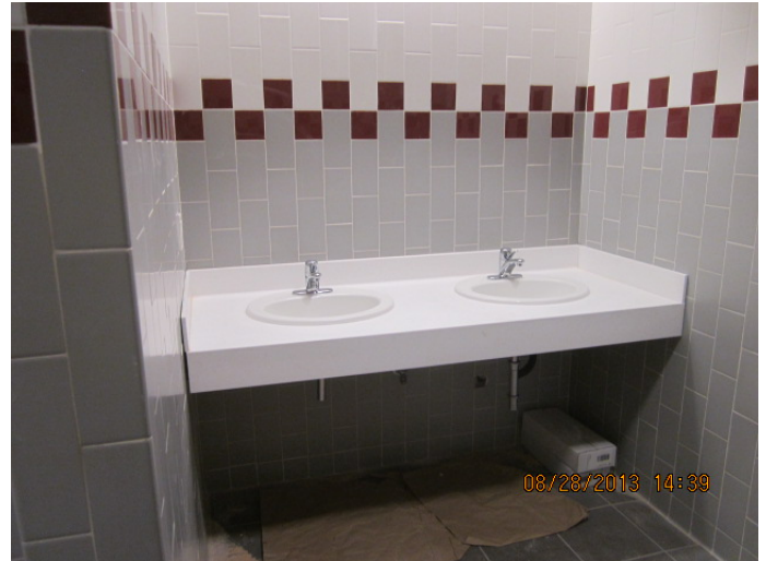
Admin. Bldg. – Tile Placement
