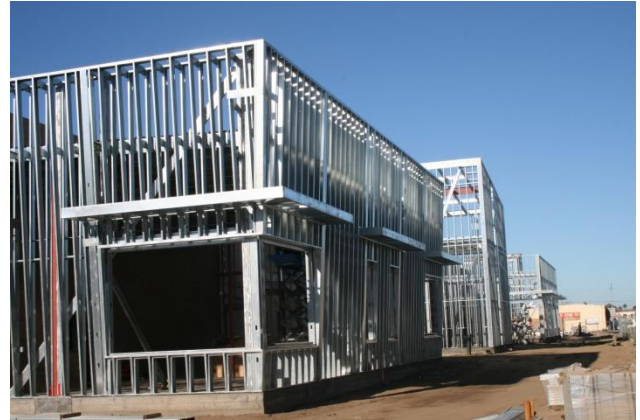
Industrial Tech Lab Building (O-200)
