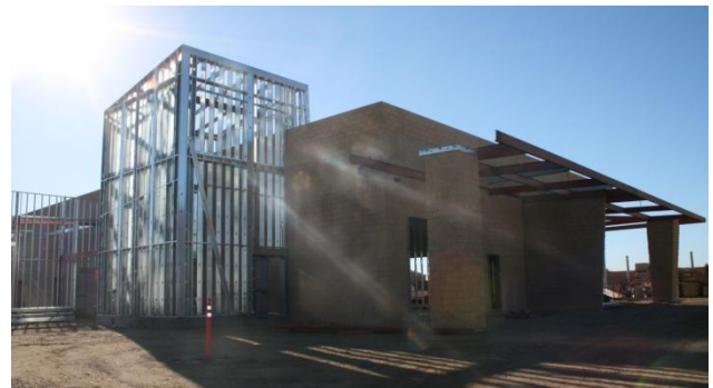
Metal Framing @ South College Drive Entrance (O-200)
