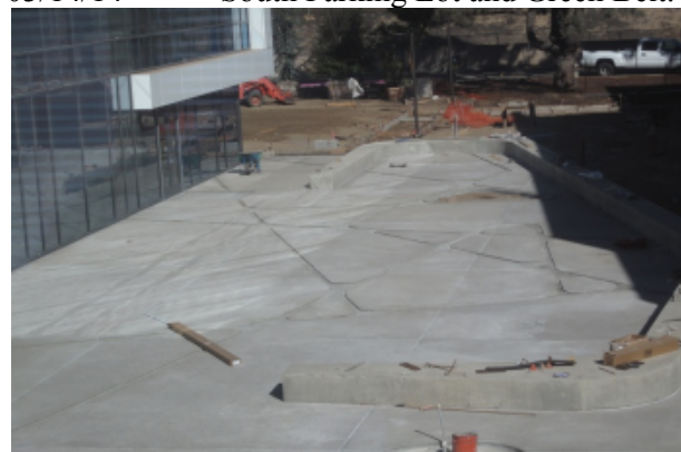
Concrete flatwork poured in center courtyard.
