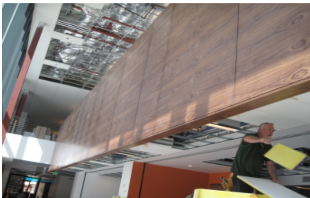
Wood paneling installed in at Info Commons Area
