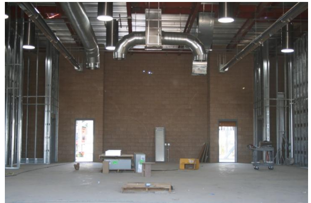
Metal Framing & Mechanical Installations @ Welding Lab (O-200)
