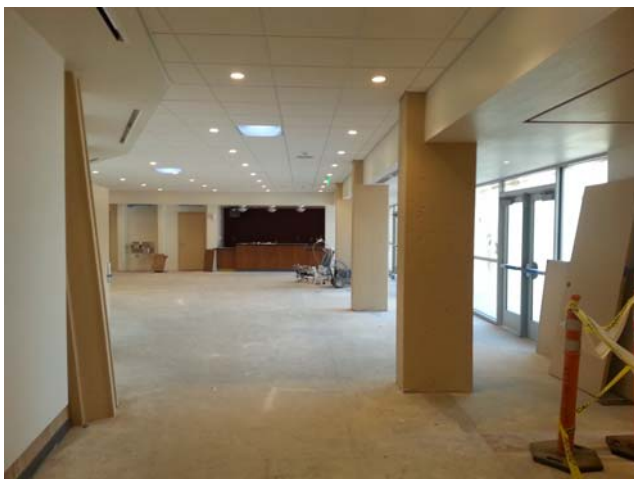
New Lights & Skylights at Lobby
