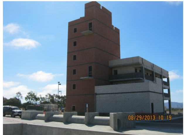
Fire Tower Bldg. –CMU completed
