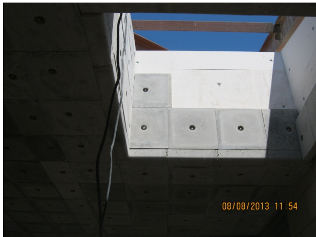
Class A Burn Bldg. HTL – Shaft wall
