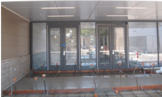
Exterior doors have been installed at all buildings.
