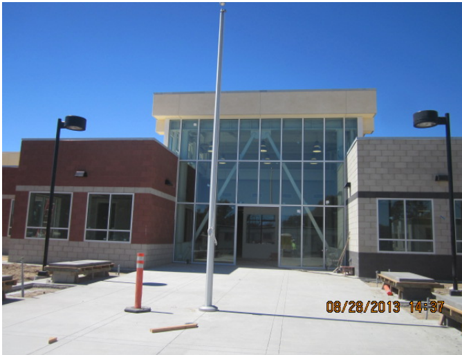
Administration Bldg. – Main entryway
