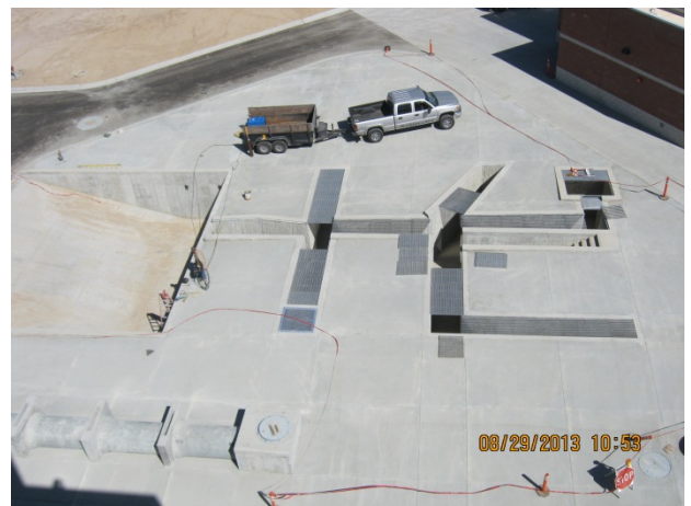
Trench Rescue – Installation of metal grids
