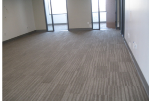
Carpet installation complete at Building A 2 nd Floor
