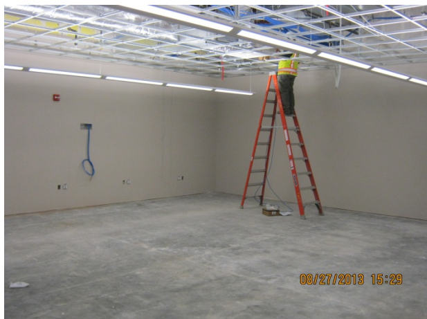
Admin. Bldg. – T-bar ceiling installation
