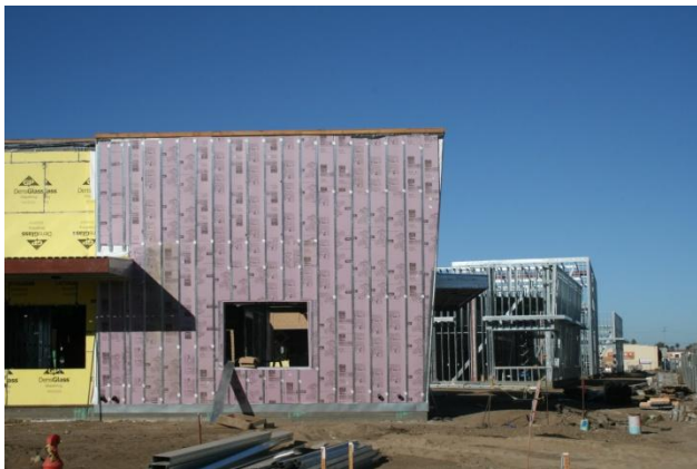
Admin. Building O-100 (O-200 Classrooms in Background)
