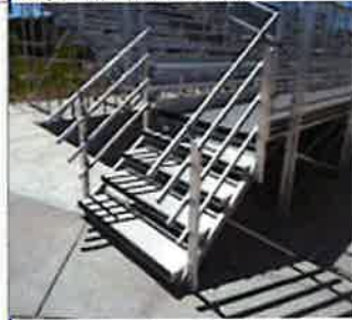
4. Staircase, Metal Handrails - Concrete Wall Below
