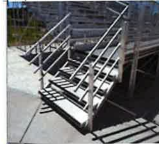
8. Staircase, Metal Handrails - Concrete Wall Below
