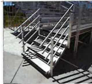
6. Staircase, Metal Handrails - Concrete Wall Below
