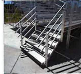
9. Staircase, Metal Handrails - Concrete Wall Below
