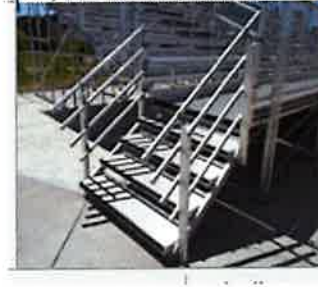
10. Staircase, Metal Handrails - Concrete Wall Below
