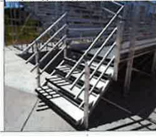
5. Staircase, Metal Handrails - Concrete Wall Below
