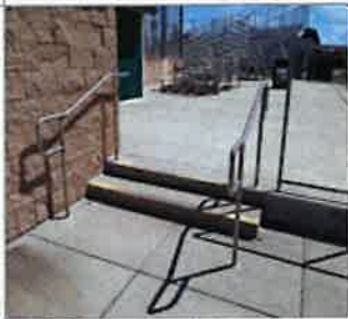
1. Staircase, Metal Handrails - Concrete Wall Below
