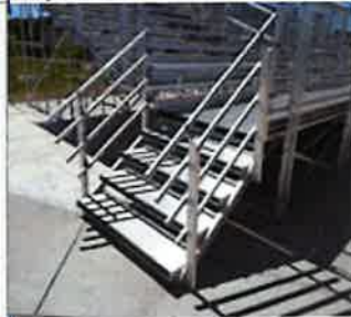
3. Staircase, Metal Handrails - Concrete Wall Below
