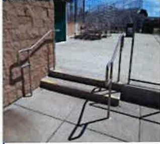
2. Staircase, Metal Handrails - Concrete Wall Below
