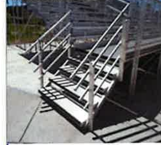
7. Staircase, Metal Handrails - Concrete Wall Below
